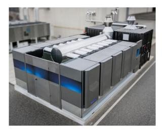
Figure 3: Bloom Energy's heat capture installations
